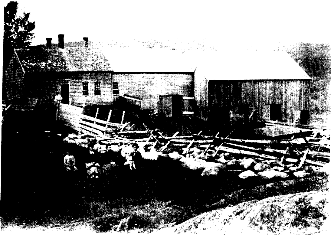
Figure 8. The boarding house for the Madison Slate Quarry workers, showing random boulders, a split-rail fence atop a field-stone base, and a sawn board fence (MHPC collection).
