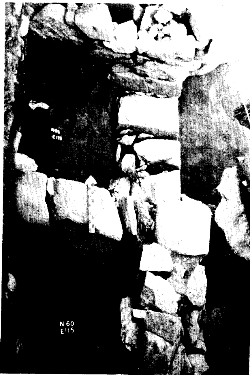
Figure 2. Photo showing remains of western wall of Halifax II. Bulkhead is in upper left quadrant, and wall of Halifax I is barely visible in upper right corner. Lower right corner is location of laid-up brick.
