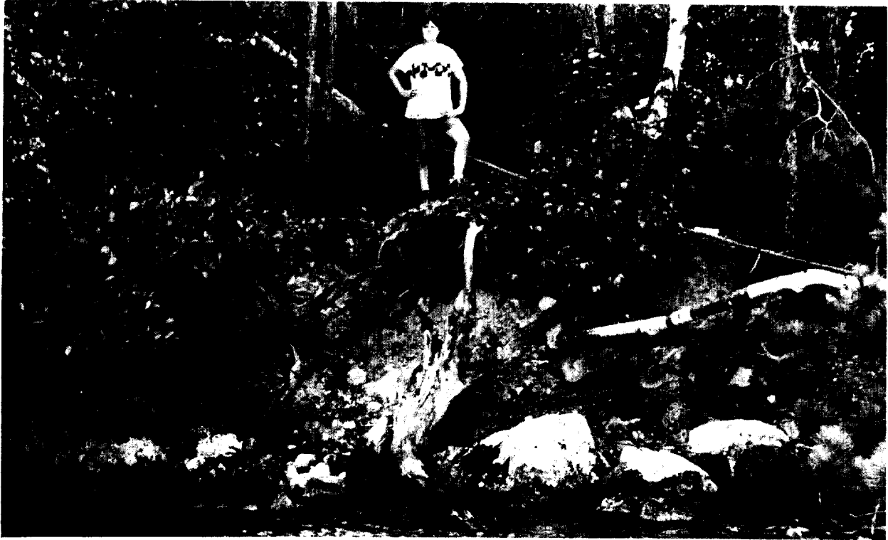
Figure 12. View of severe erosion at site ME 37-18 in the Oakland Project area, facing north. Note crew member for scale.
