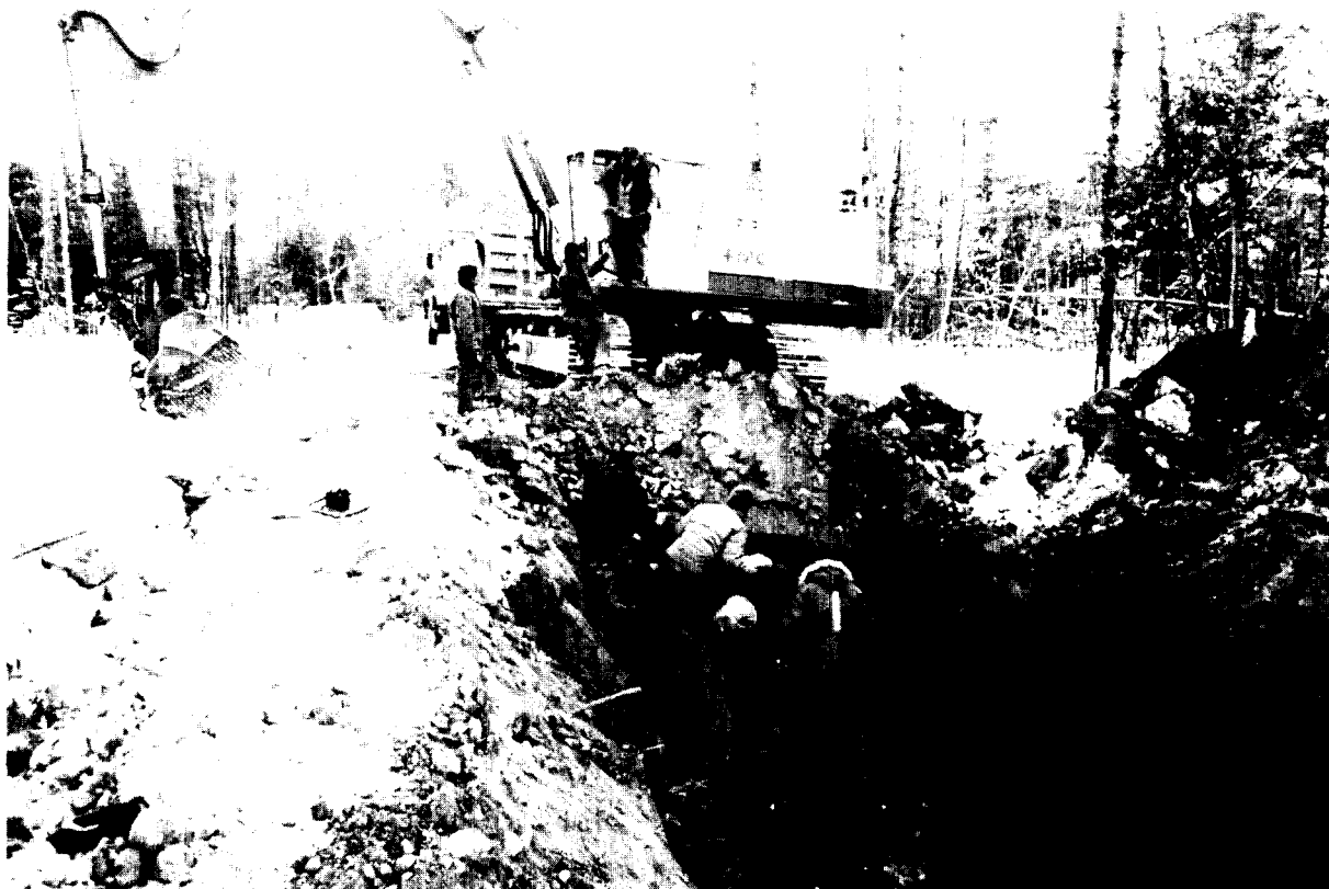
Figure 5. Overview of UMF archaeologists salvaging cultural feature exposed in large construction trench, facing west, January, 1989.
