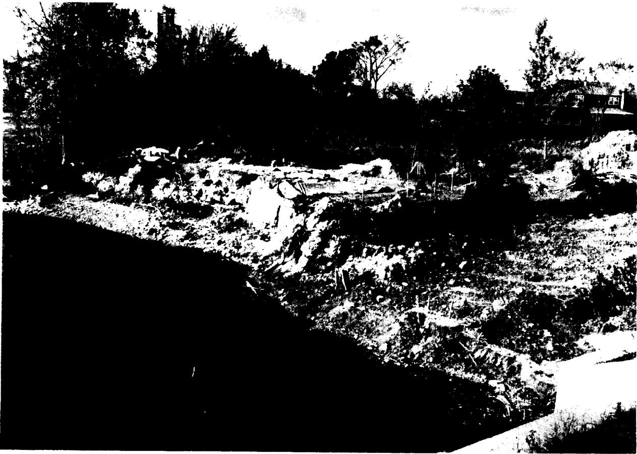
PLATE 2 Two kinds of excavation in progress. In the foreground is the excavation for new culverts; beside it is the archaeological project.
