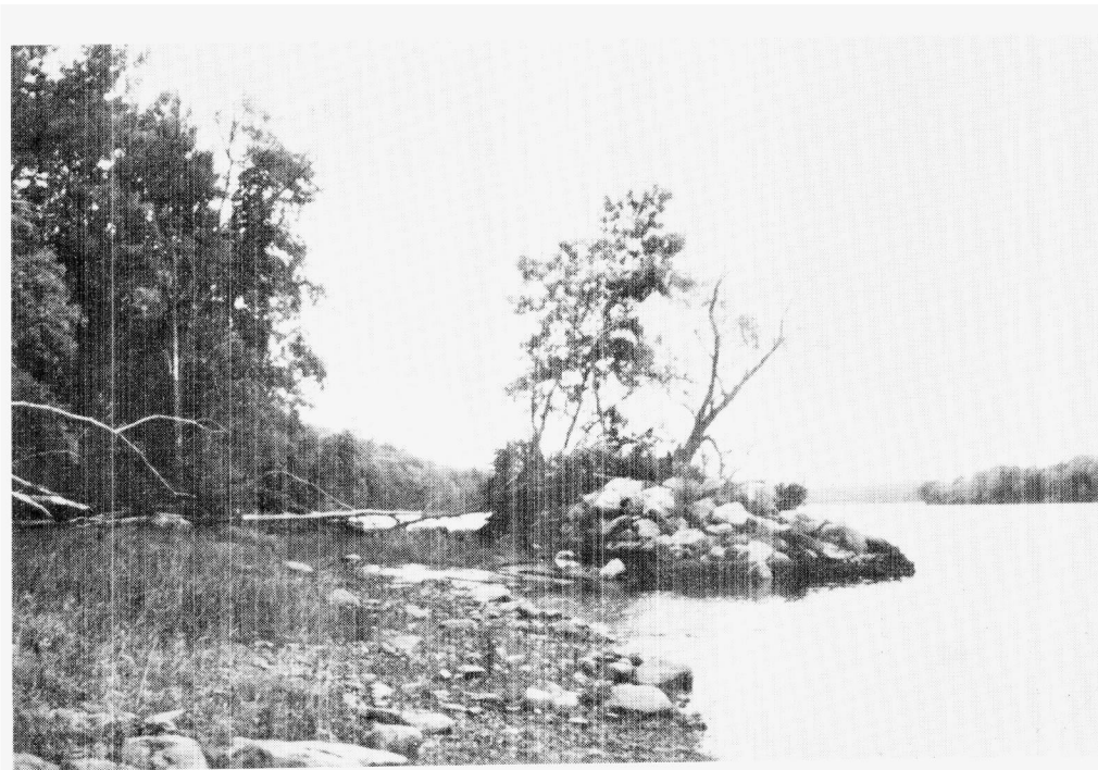
Figure 2. Ice House Features. Top : Lower of two cisterns supplying steam engines. Bottom : Best-preserved of two shipping piers. (Photos by Peter Lund, printed by UCPS.)
