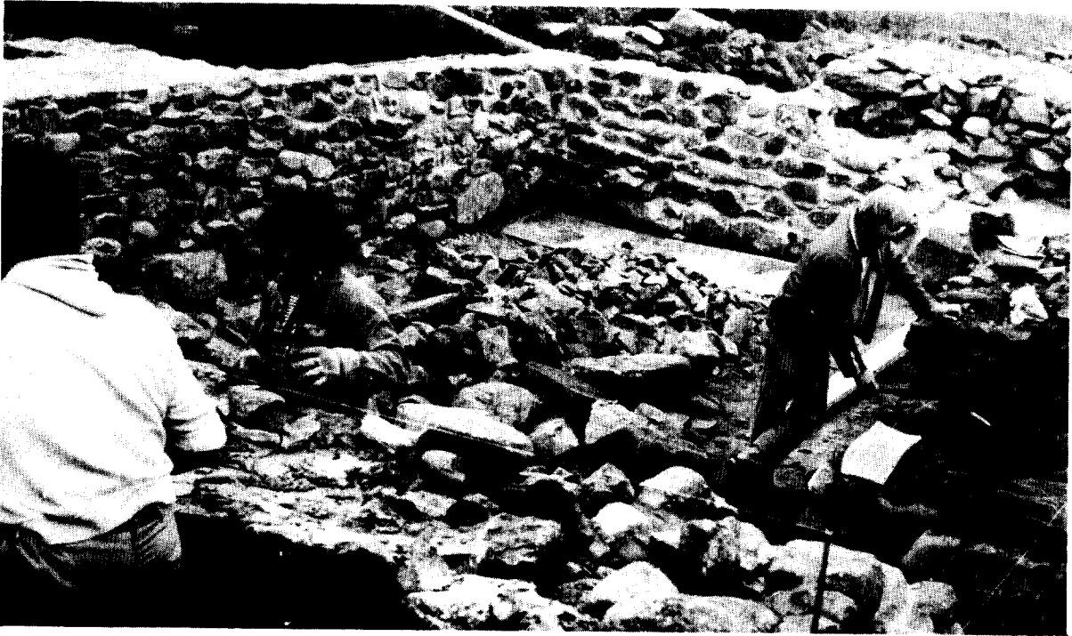
Above: Stabilization in progress; wall excavation (right), wall mortaring (left), completed treatment (rear). Below: Stabilized features in January, with Fort House beyond.
