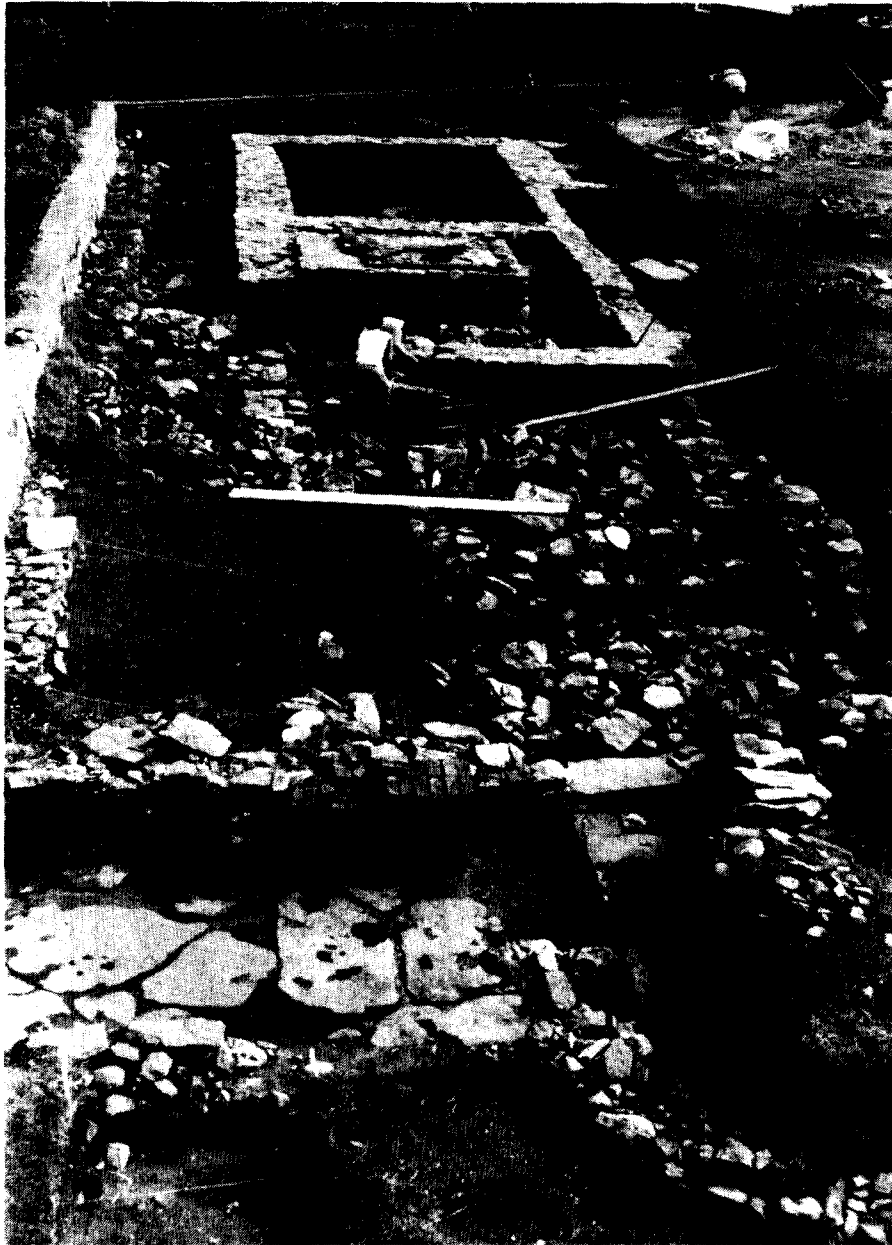
General view of project. Background structure stabilized. Foreground: paved rear entrance of 1692.
